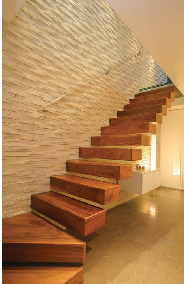
Cantilevered walnut clad treads with stainless steel handrail.
