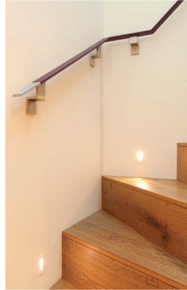
Schottenhansen oyster oak treads and leather wrapped stainless steel handrail.
