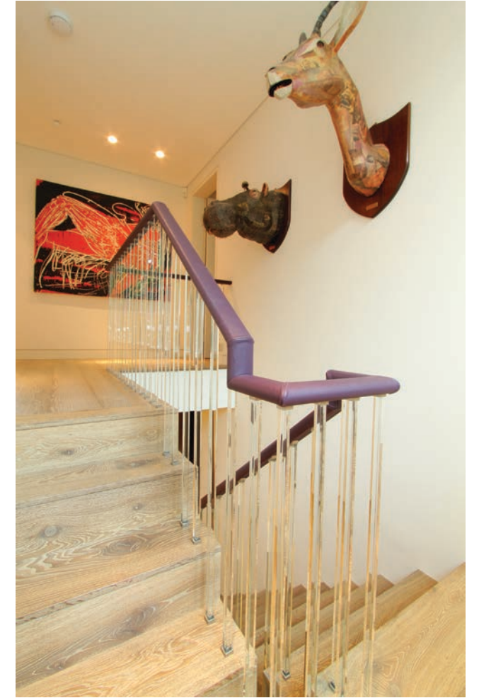
Schottenhansen oyster oak treads with square glass spindles and leather wrapped handrail.
